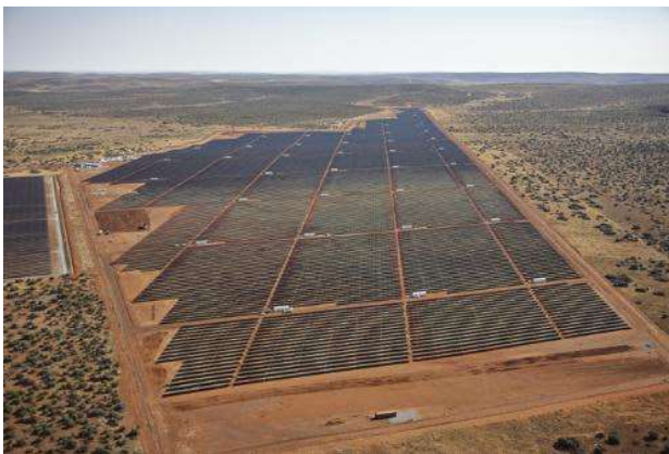
Typical PV Plant
