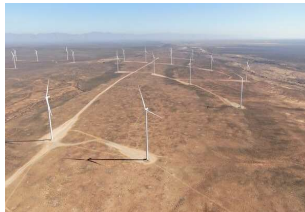
Typical Wind Farm
