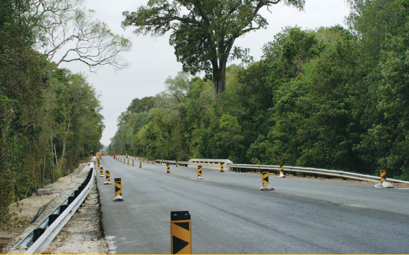
A 20 metre span two metre high bridge was constructed to protect the roots of a 500 year old yellowwood tree growing alongside the recently upgraded N2 highway between Tsitsikamma and Witelsbos
