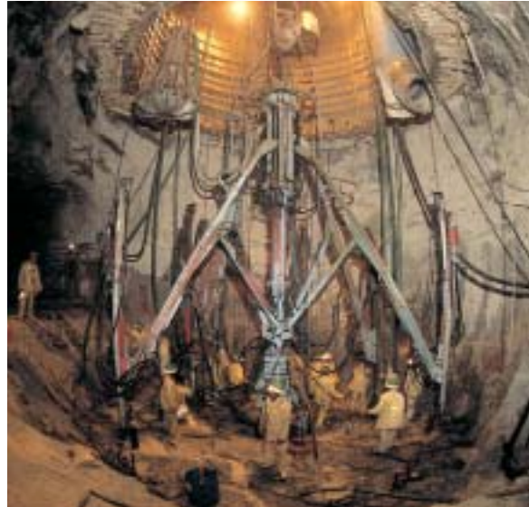
Shaft sinking and equipping
