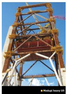
A major lift of 1 160 tons undertaken in July 2010 to erect the roof of the first Medupi boiler used a method called strand jacking to ensure the highest levels of precision and safety. The process involved the lifting of a heavy steel grid that will house the boiler onto a 104 metre high steel frame.
