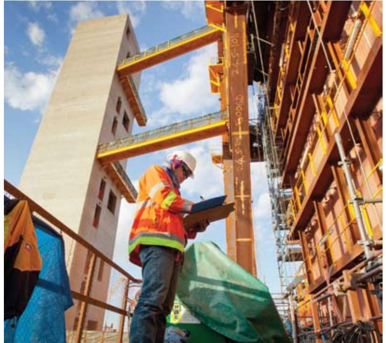
4 Medupi power station under construction
